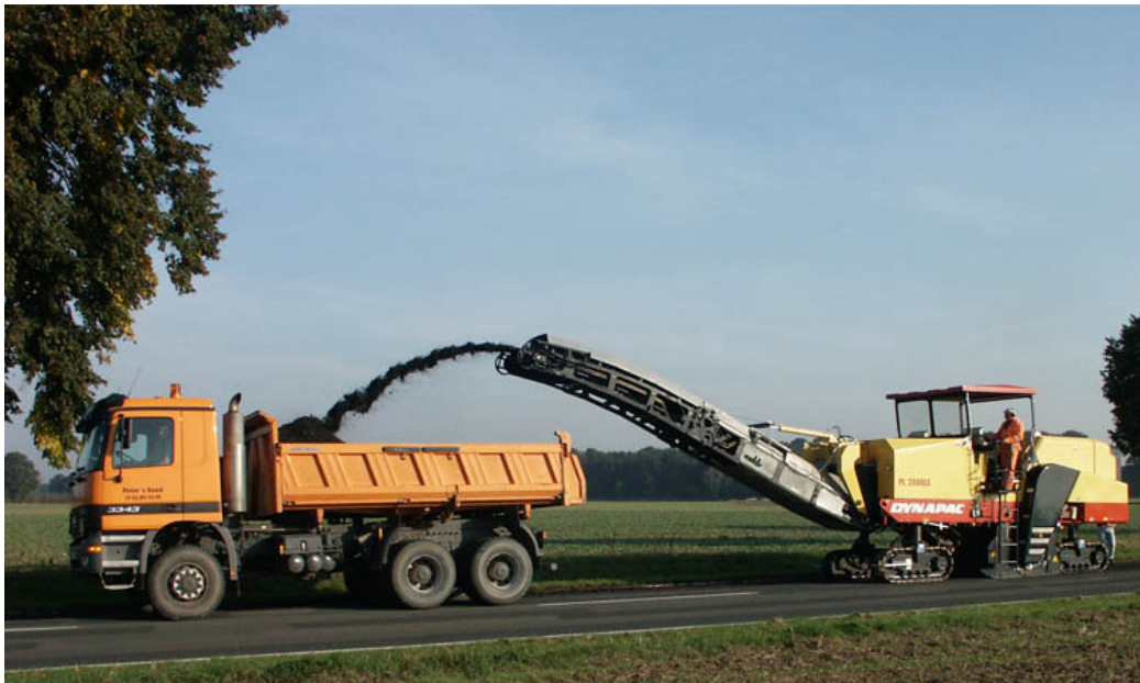
Figure 3 A planer and a truck in action, planing off old asphalt.
